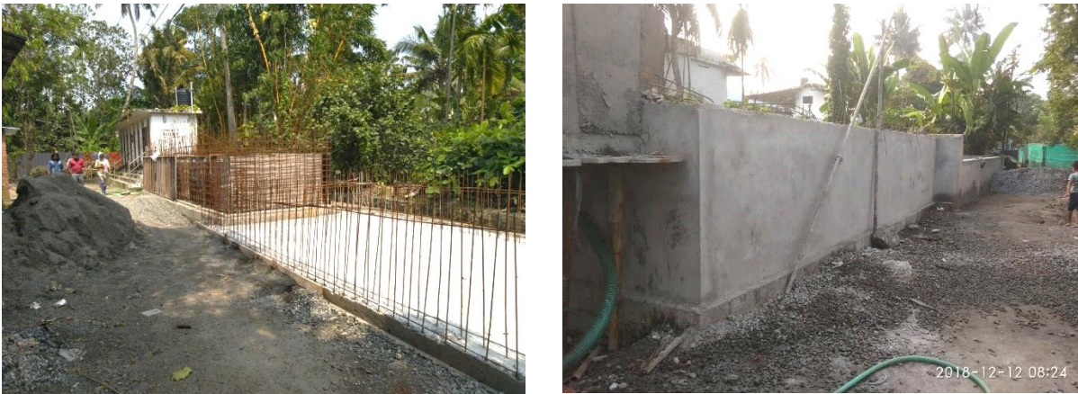
Figure 8.2 Under construction community DEWATS system in Municipal colony
