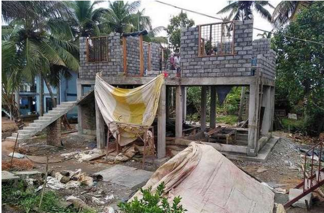
Figure 8 : Typical Under-Construction House on Pillars in Kainakary, Kuttanad (Paul, 2019)
