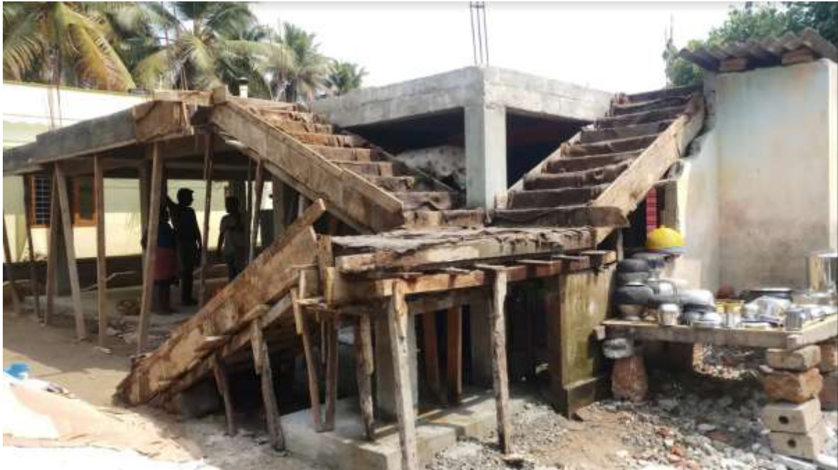
Figure 51: Under construction Frame structure on Stilts in Kainakary, 2019
